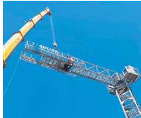
Fast installation of the boom
